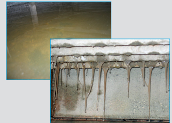
Flour & Yeast make glue in condenser. Bacteria count exceeds 1,000,000 CFU/ml
