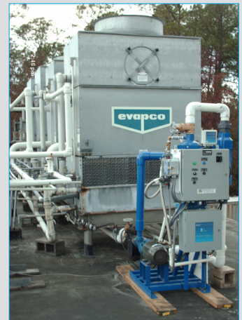
Griswold treatment cleaned the system and reduced bacteria to less than 1,000 CFU/ml
