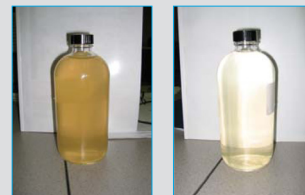
Chilled Water Before and After
